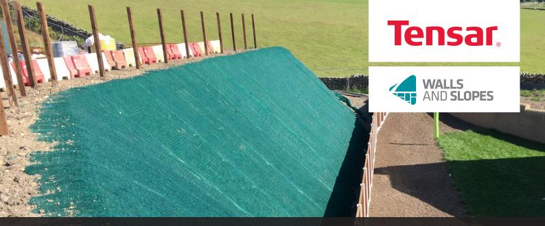
The reinforced soil slope was used to maximise space for homes and gardens at two levels on the sloping site.
